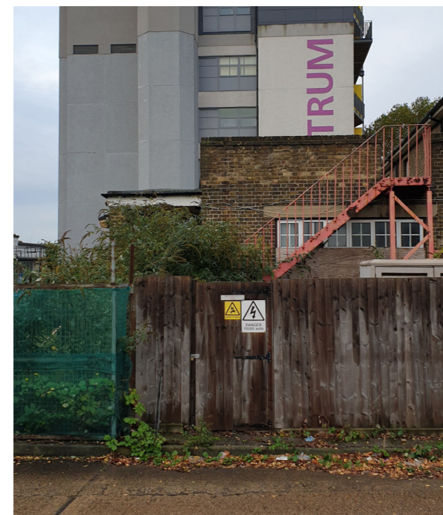
5. Dilapidated buildings with residential building in background
