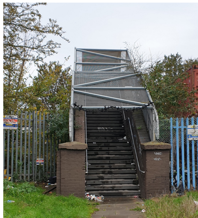
4. View from Footbridge (north)
