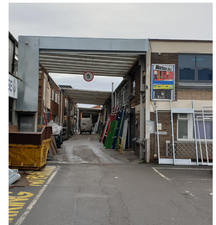
6. Existing building fabric of many units is dated
